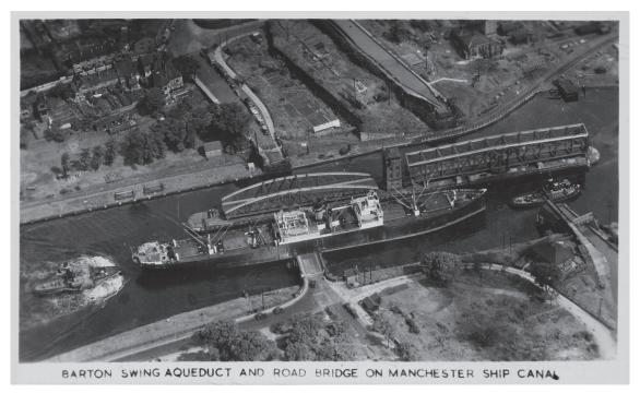
The photograph shows the first and only swing aqueduct in the world. In this picture it has been swung open to allow the passage of a ship heading towards Manchester. The Barton swing aqueduct was just one of the many engineering feats that enabled Victorian entrepreneurs to turn Manchester, a city which is 64 km inland, into Britain's third largest port.
