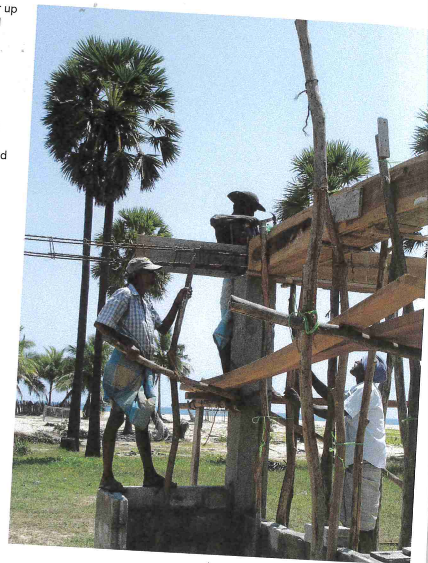
△ Construction of community infrastructure, including a fish market (shown here).
