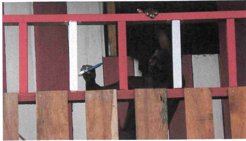
△ Community members paint new infrastructure.
