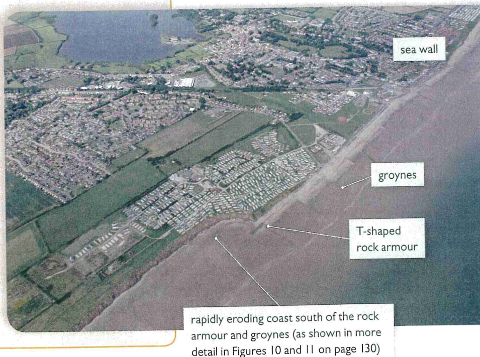
Figure 9 Hornsea – coastal defences
