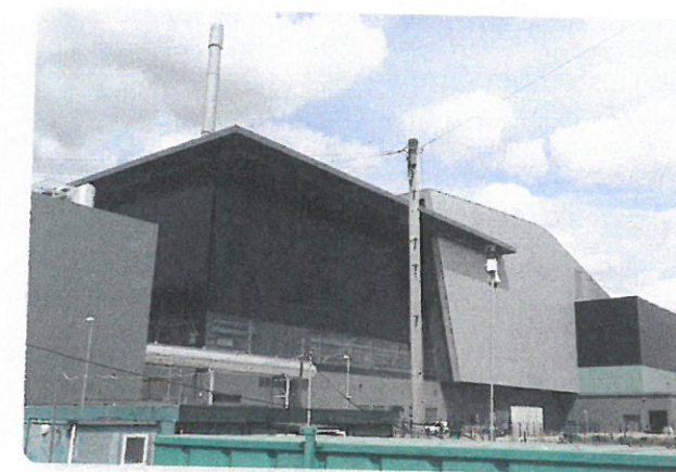
▲ Figure 8 Lincolnshire's Energy from Waste facility, North Hykeham, Lincoln
