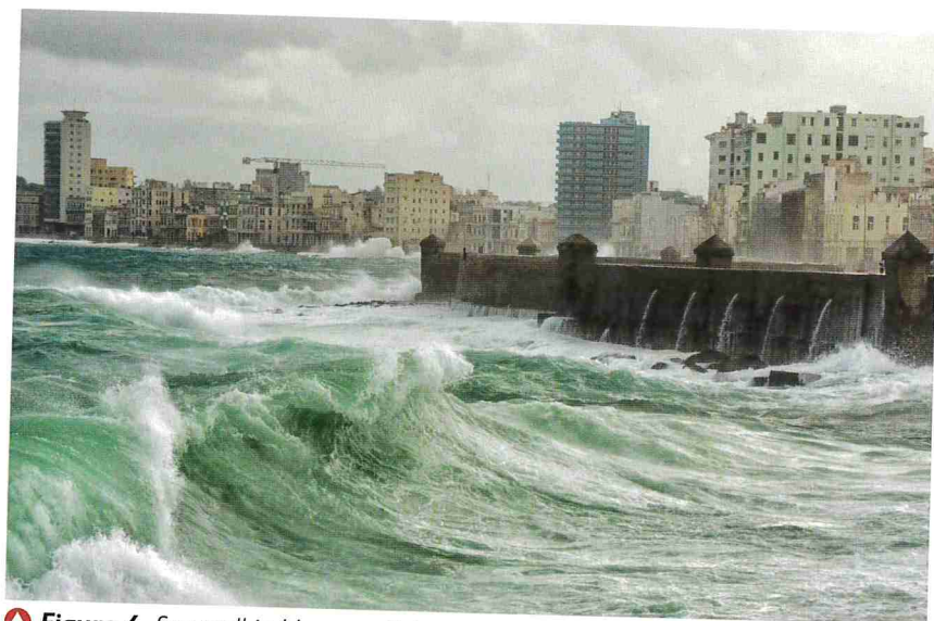
Figure 6 Sea wall in Havana, Cuba protecting the city from storm surge
