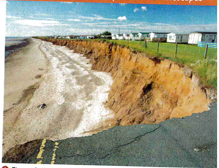
Figure 3 Recent erosion threatening the settlement of Skipsea, where rates of erosion are 2 metres a year
