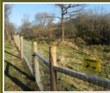
The 900 m perimeter fence has electric strands to prevent beavers climbing and a weldmesh apron on the inside to prevent them burrowing underneath. This fencing cost approximately £35/m to construct.
