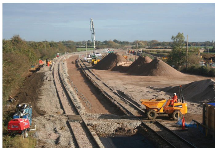
Photo. 2 Construction of the new dual lines
