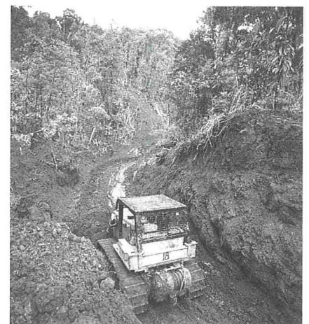
The building of new road networks into regions with tropical rainforests causes considerable environmental damage. In areas with very high rainfall there is an increased risk of erosion and loss of topsoil.
