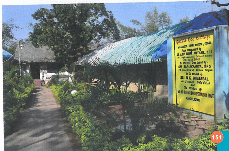
▼ Figure 8 Godwit Eco Cottage is a collection of holiday cottages close to Chilika Lake. They are made of bamboo and mud, with thatched roofs.
