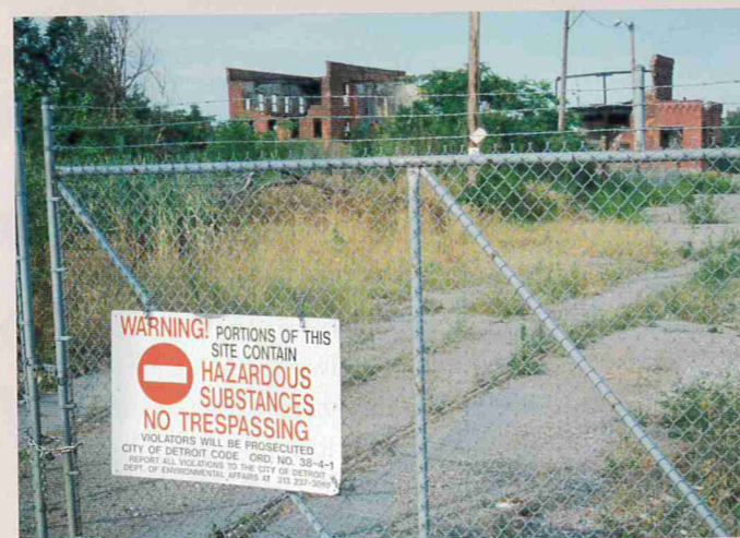
Figure 8 'If you come here at night it glows.' The Uniroyal tire plant closed in the 1980s, forming part of the drosscape of Detroit. In 2012, the first step in revitalising Detroit's waterfront began, including the excavation of this site to a depth of nine metres.
