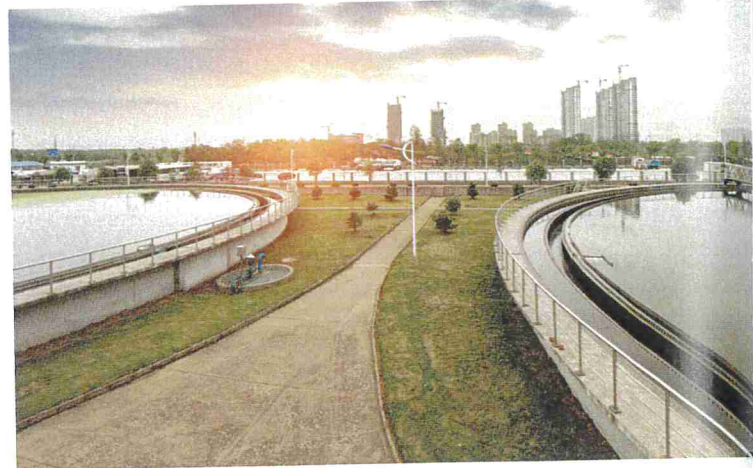
✓ Figure 1 Modern urban waste water treatment
