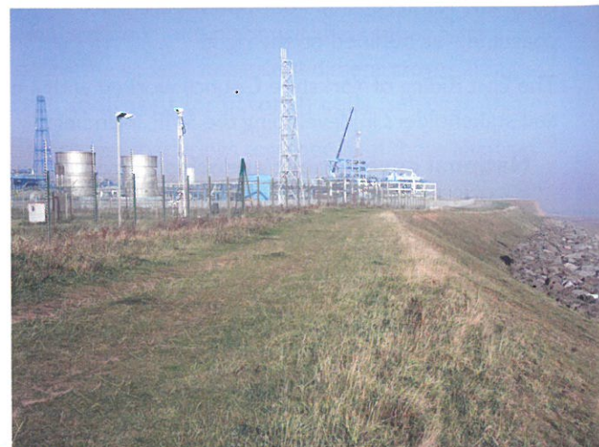
▼ Figure 3 Easington gas terminal is protected by a rock revetment
