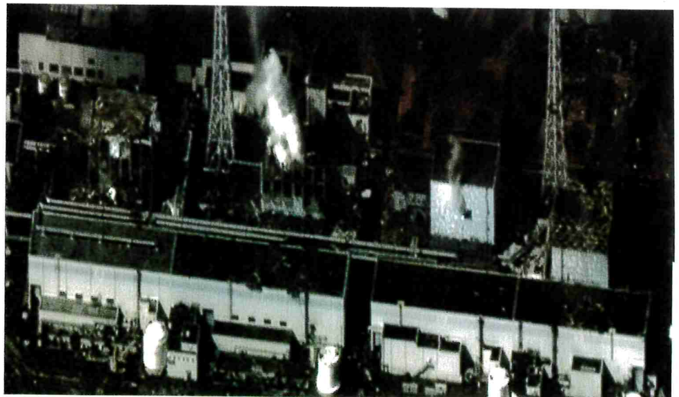
Figure 4 The Fukushima Daiichi nuclear power plant after the earthquake and tsunami. Reactors 1 to 4 are from right to left. Three of these reactors overheated, causing meltdowns that eventually led to explosions releasing large amounts of radioactive material into the air.
