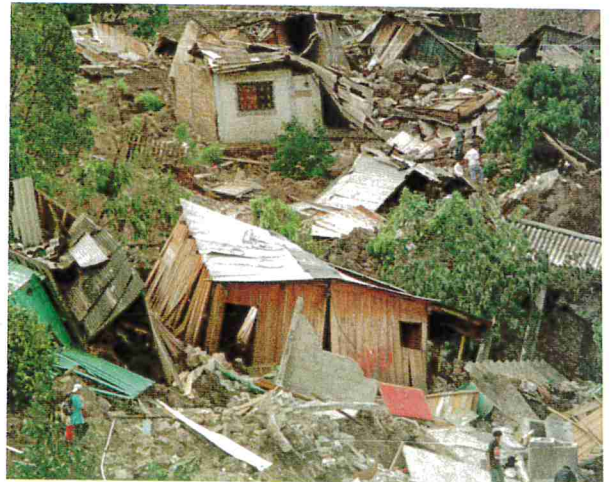
Figure 8 Landslide caused by Hurricane Mitch, 1998
