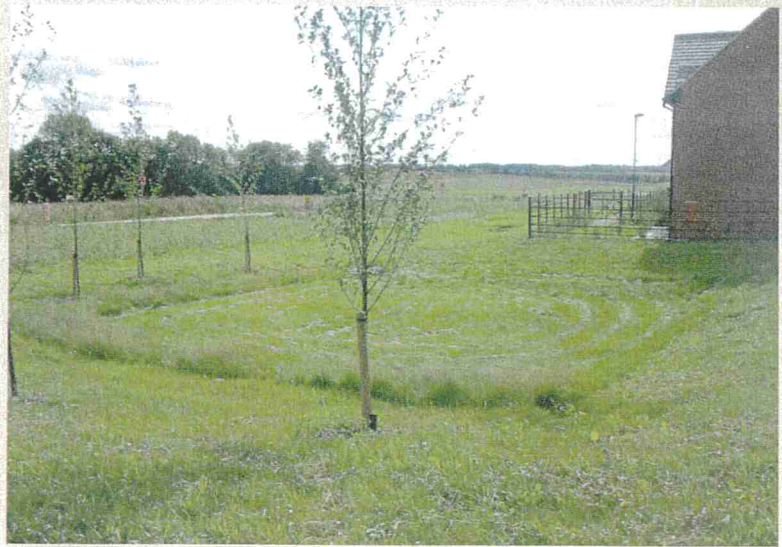
Figure 4 Detention basin, Lamb Drove, Cambourne
