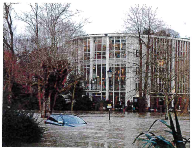
▲ Figure 3 Torrential rain and hail caused the River Wey to burst in banks in Guildford, December 2013
