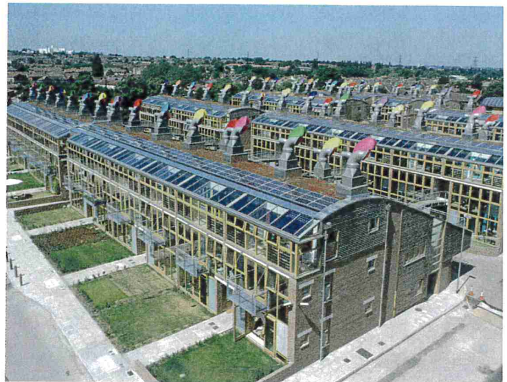
Figure 3 BedZED consists of 82 'affordable' homes, 18 workplaces, retail and leisure areas. It includes a children's nursery, medical centre, sport pitch, exhibition centre, offices and meeting rooms. The scheme includes a biomass-combined heat and power plant, an onsite sewage treatment and rainwater recycling system, and natural wind driven ventilation.
