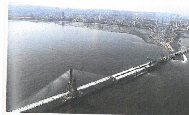
Figure 9.70 Mumbai's skyline resembles that of a wealthy city. The Bandra-Worli Sea Link shown in the photo is a cable-stayed bridge that connects central Mumbai with its western suburbs.
