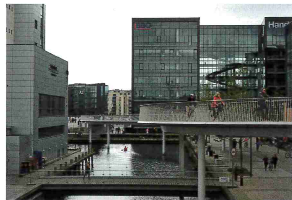
Figure 9.62 The elevated Cykelslangen , or Cycle Snake opened in Copenhagen in 2015. It is a two-way 220-metre bridge. You can get across the harbour in less than a minute, creating a less stressful atmosphere for cyclists, pedestrians and vehicle users alike
