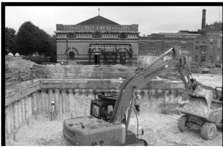
Figure 2: Foundations being dug
