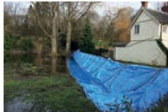
A flood barrier to protect a house from river flooding
