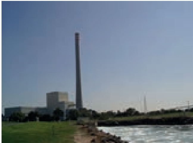
► Power station hot water discharge
