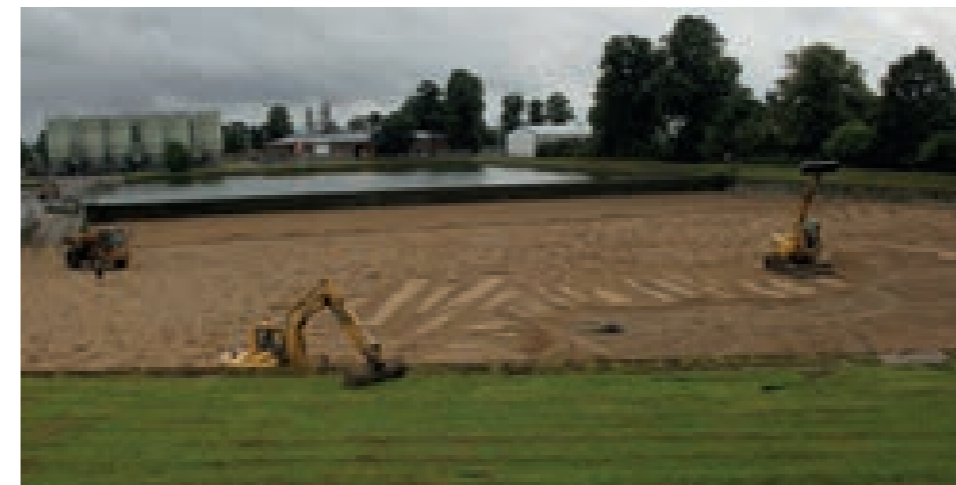
▲ A sand filter being constructed
